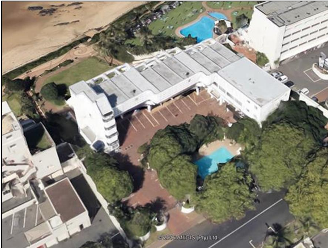
Figure 1: An aerial view of the existing structure of the “Fleetwood on sea” hotel located on Lagoon Drive.
