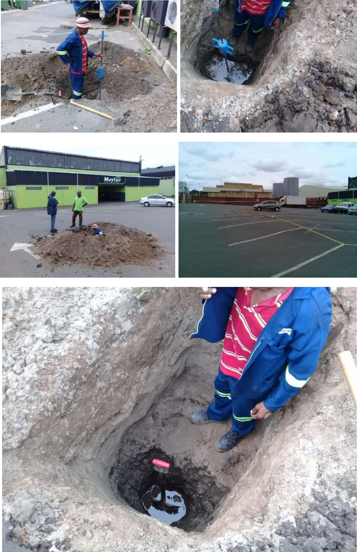
Figure 23: A collection of site photos showing fieldwork.
