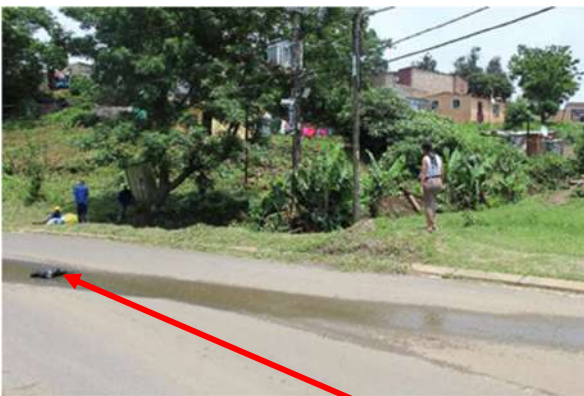
Plate 7: The proposed pipeline will cross the road at 29° 43' 18"S; 30° 55' 01"E.
