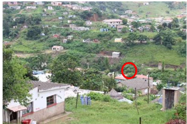
Plate 8: The reticulation to tie-in to the existing pipeline (circled in red)
