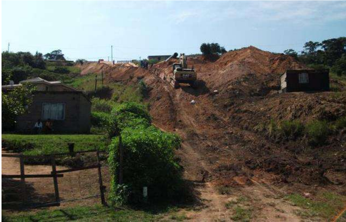
Figure 7: Excavations for water pipeline
