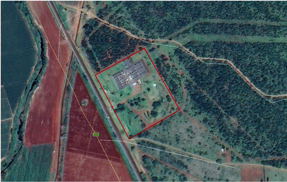
Figure 6: Aerial Snapshot of the Existing Pongola 132 / 22kV Distribution Substation (Google Earth Image, 2018)
