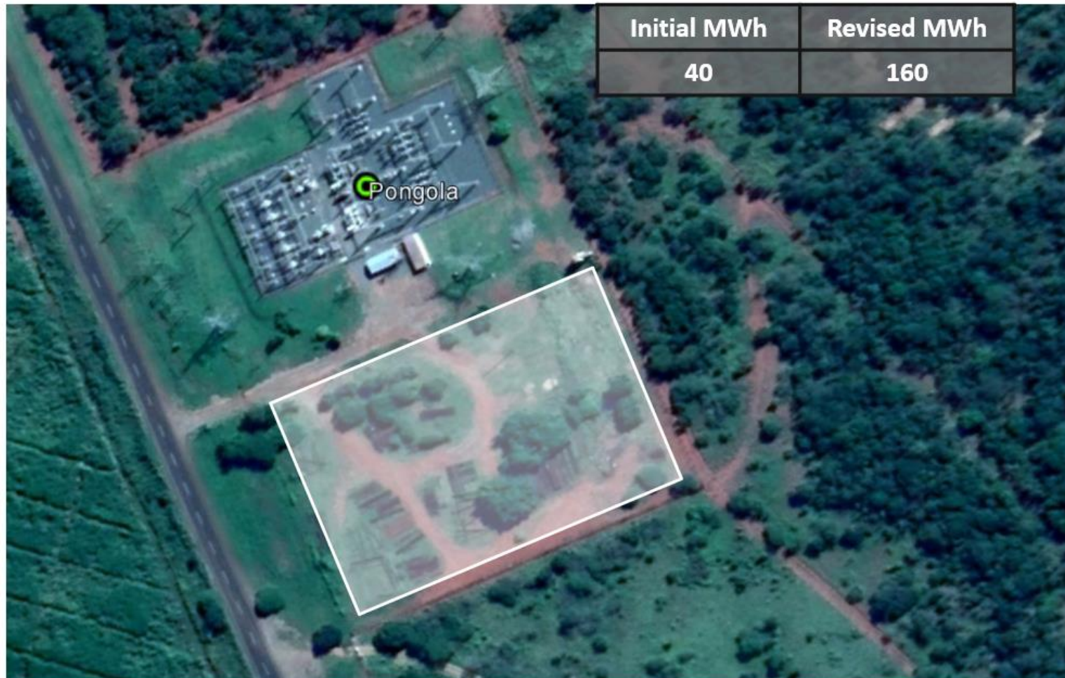
Figure 3: Pongola Substation and Proposed Area for BESS (white), (Eskom, 2019)
