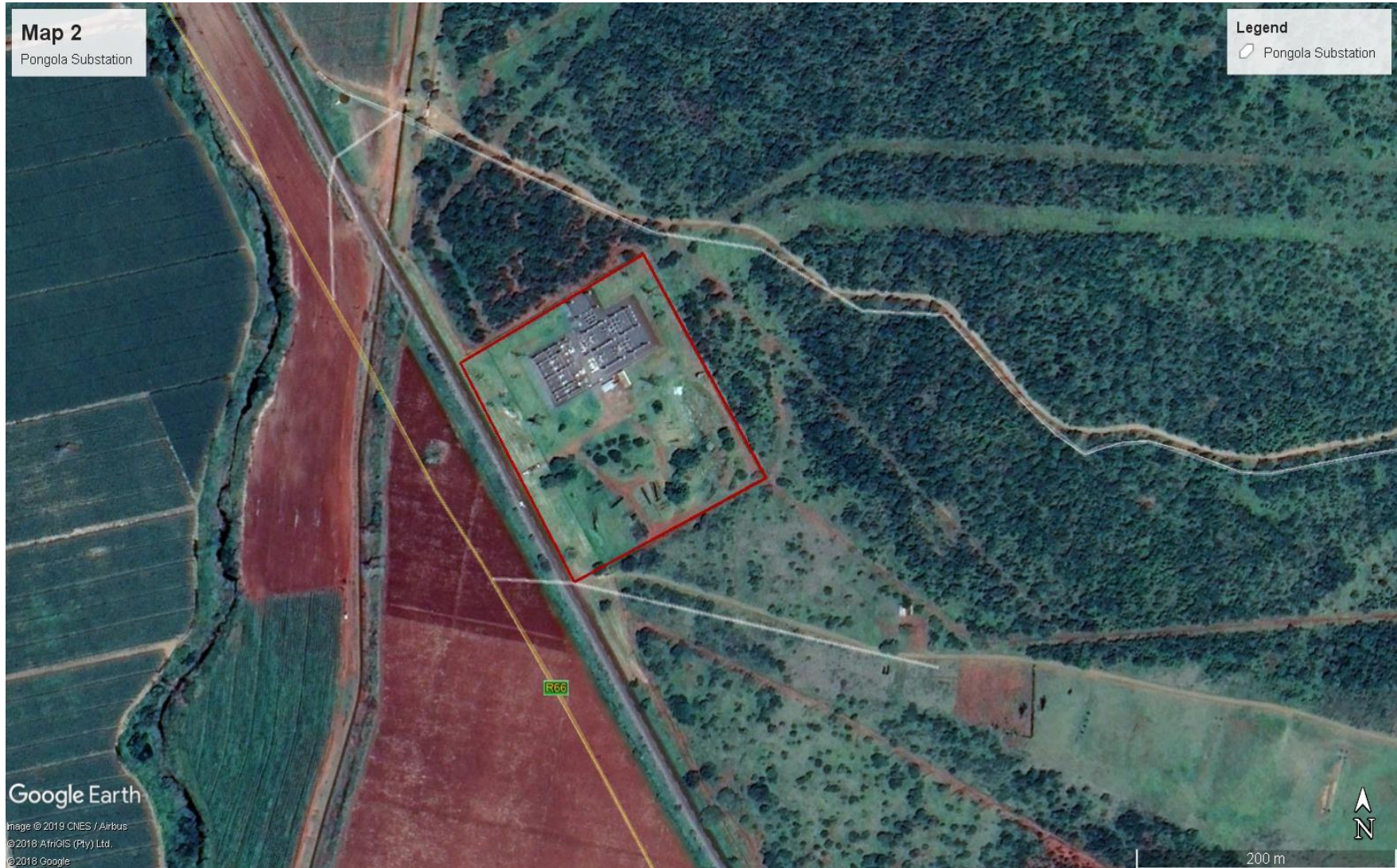
Figure 2: Pongola Substation (Red), (Google Earth Imagery, 2018)
