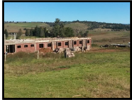
Plate 8: North West View of the site
