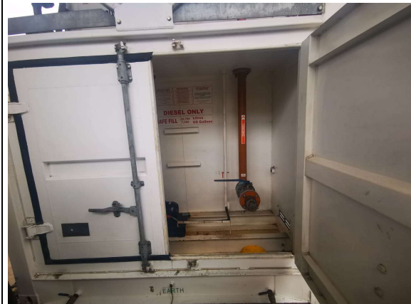
Plate 4: Opening of aboveground self-bunded diesel storage tank
