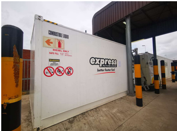
Plate 3: 28 750 litre diesel storage tank
