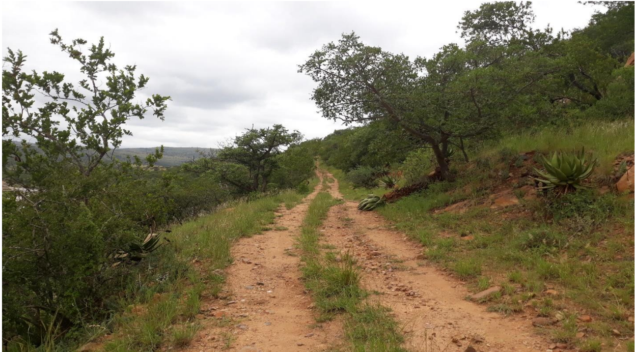
Image 2.5: Access track to the existing causeway along steep cliff face with sensitive vegetation
