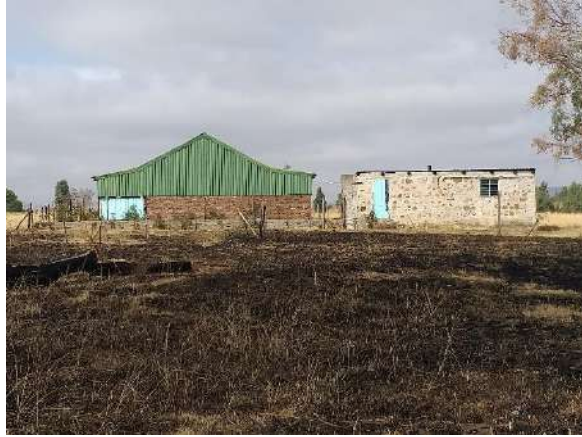
Historical structures at Wf-001
