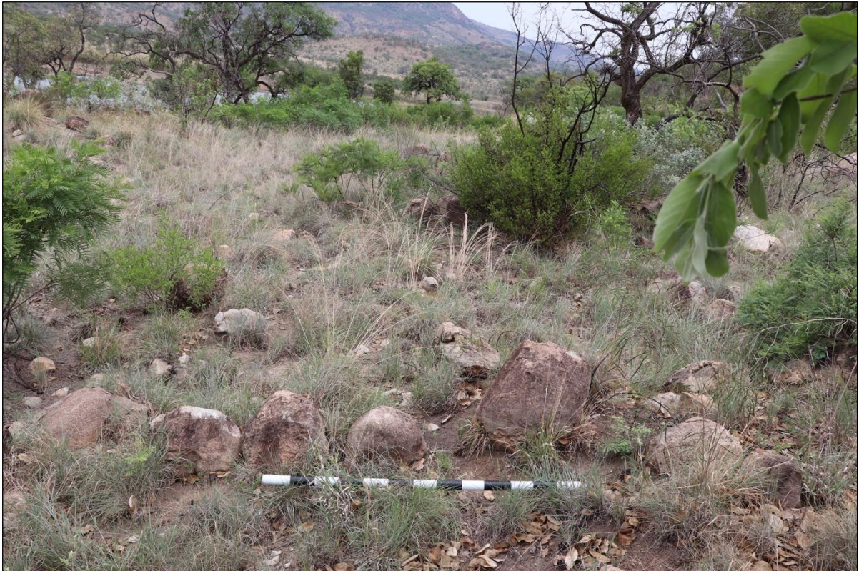
Figure 27 – General view of a section of terrace walling from site DBAP 1. The Der Brochen dam is visible in the background. Scale in 10cm increments.
