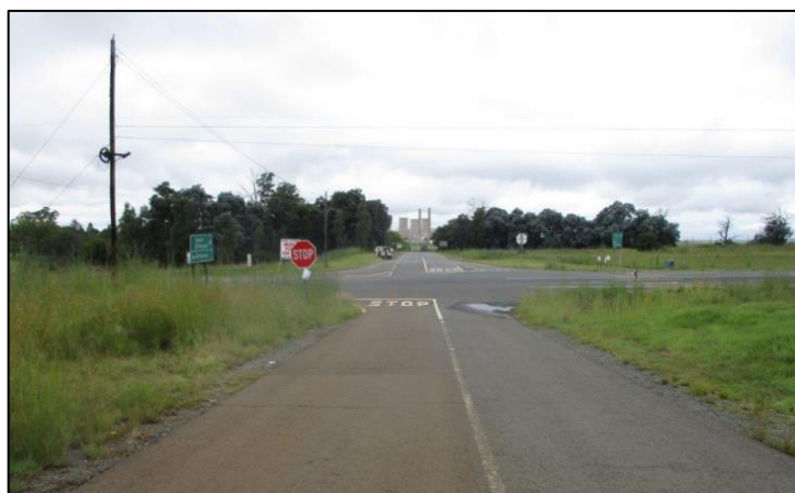
Figure 4-43: The Access Road (Road A).
