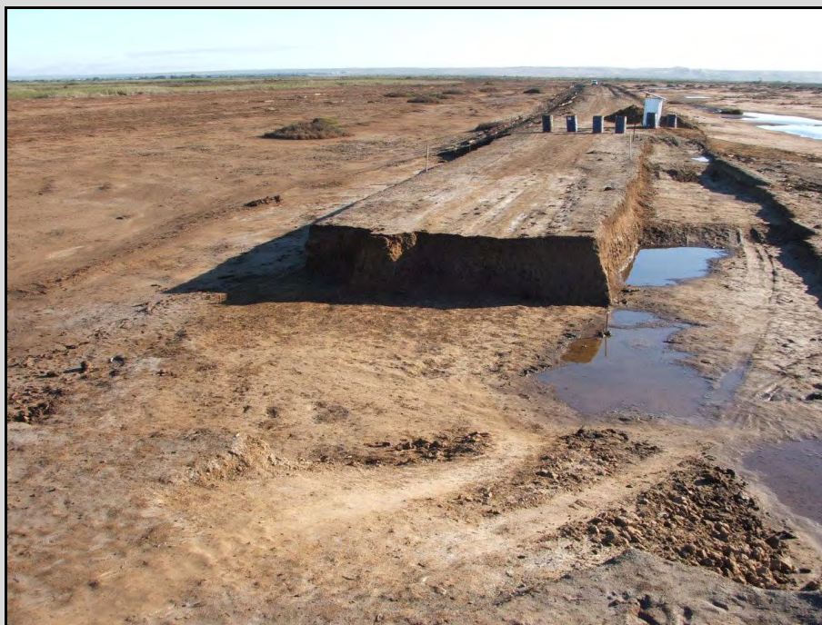
Photograph 1: An example of a break through the causeway allowing water to flow into the desertified marsh from the main Orange River channel.
