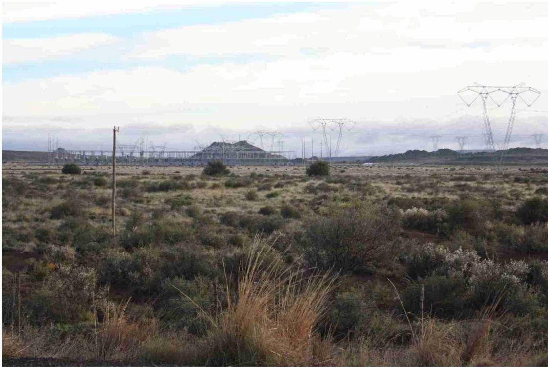
VIEW A: VIEW TOWARDS GAMMA SUBSTATION
