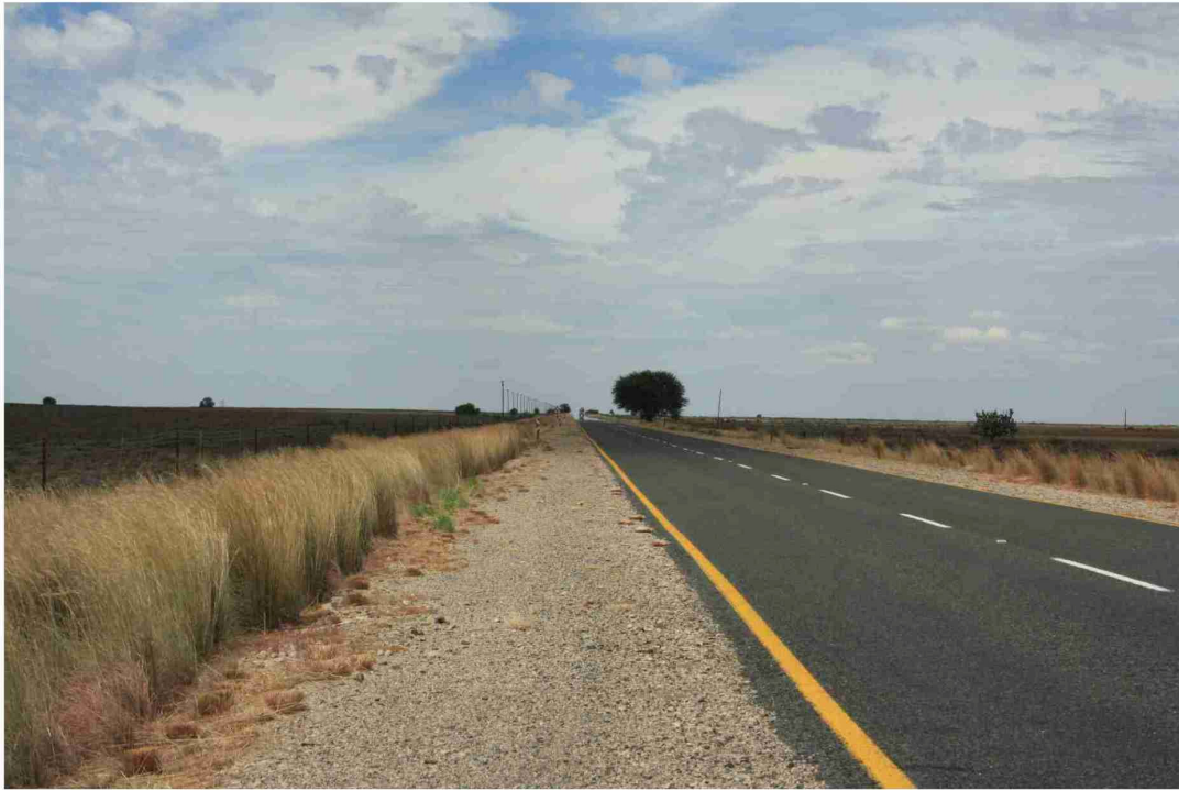
VIEW M: VIEW FROM THE R61 TOWARDS ALTERNATIVE 2
