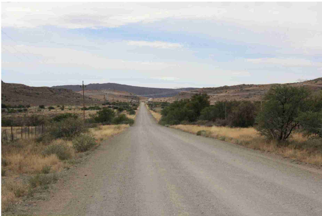
VIEW J: VIEW FROM A LOCAL ROAD TOWARDS ALTERNATIVE 2
