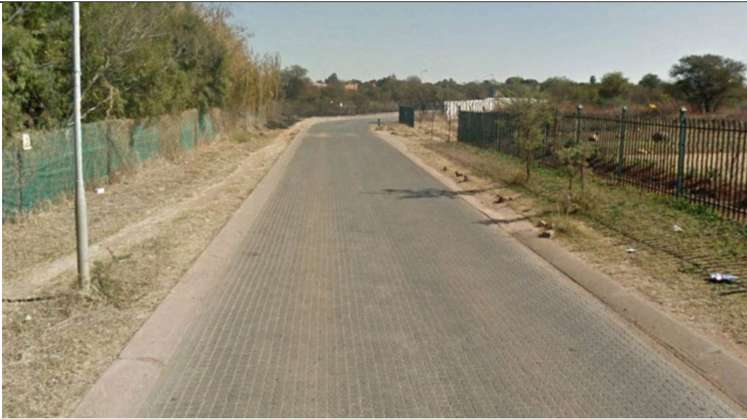
Photo 1: Existing Tsamma Street
