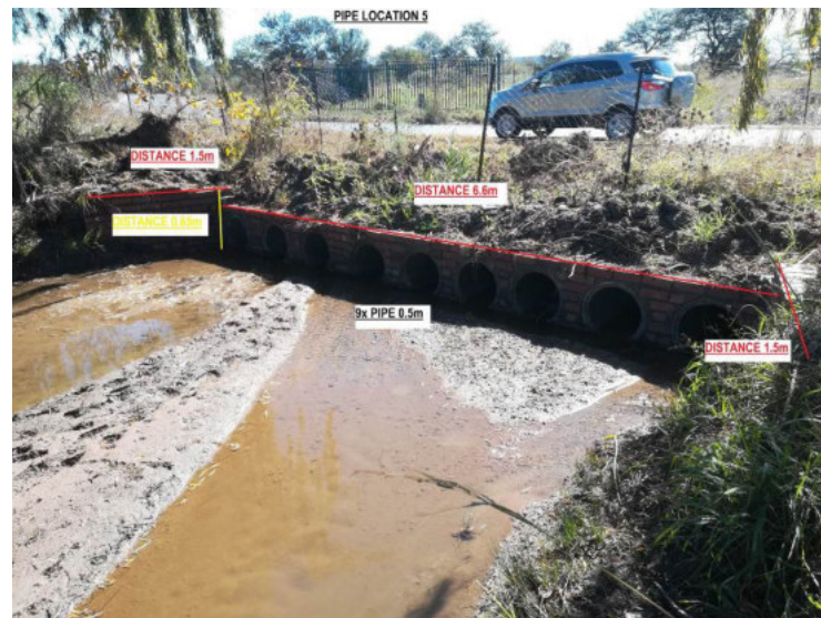
Photo 7: Existing stormwater crossing at Tsamma Street
