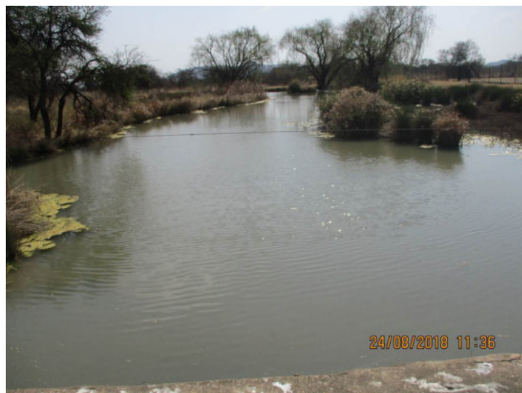
Photo 6: Existing stormwater dam north of Tsamma Street
