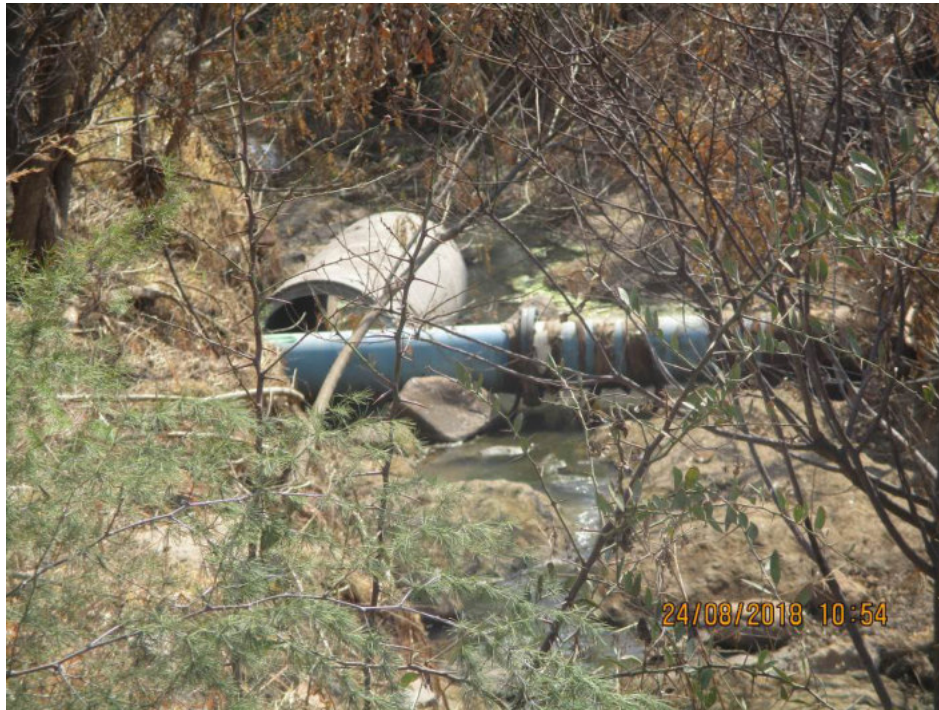
Photo 2: Existing 400Ø Steel water pipe that crosses Montana Spruit
