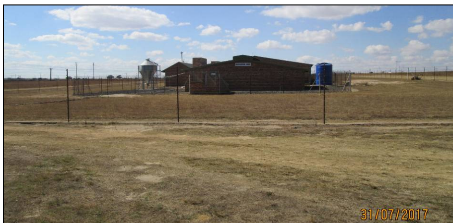
Photo 3.1: A view of the existing GTC facility located on the farm Rockdale.
