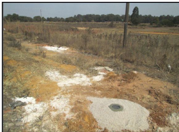
Photographic view of the newly drilled monitoring borehole
