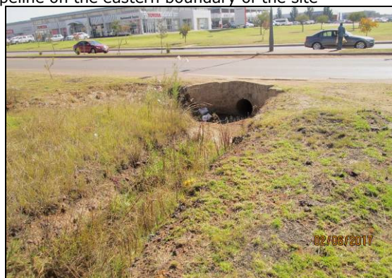
Photo 5.5: A view of the storm water culvert underneath La Roca Boulevard
