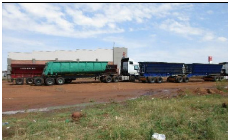
Photo 5.7: A view of the cleared western and central portions of the site.
