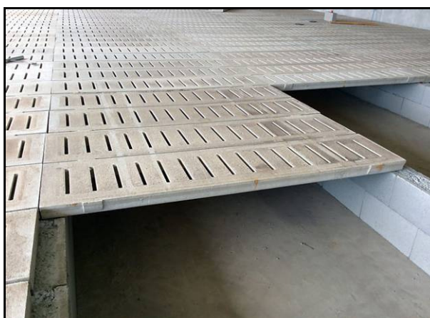
Photo 7.2: Example of the slotted floor system (obtained from www.stockyardindustries.com ).
