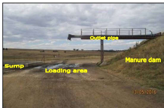
Photo 7.7: An example of the manure loading area and sump.
