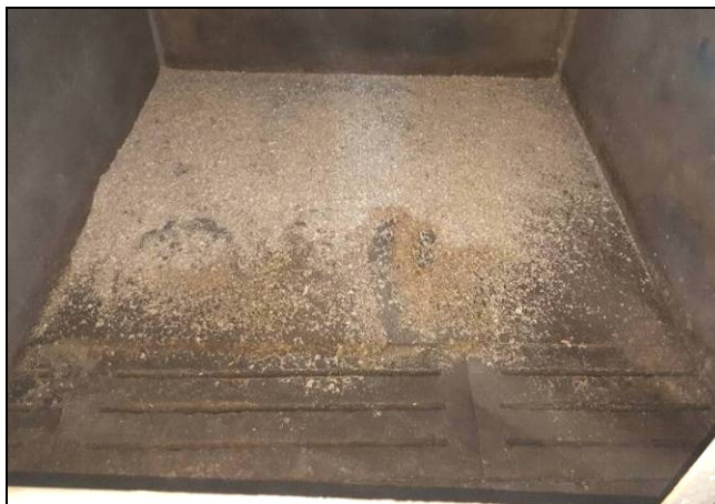
Photo 7.1: Photographic view of the concrete floor and flush channel system at the existing GTC facility.
