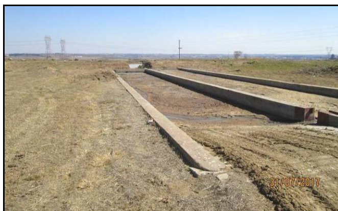
Photo 7.3: A view of the two evaporation manure pits at the existing GTC facility.
