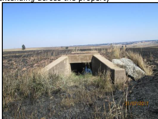
Photo 5.3: Culverts under the railway embankment
