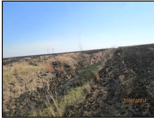
Photo 5.4: The deep trench/cutting for the railway line
