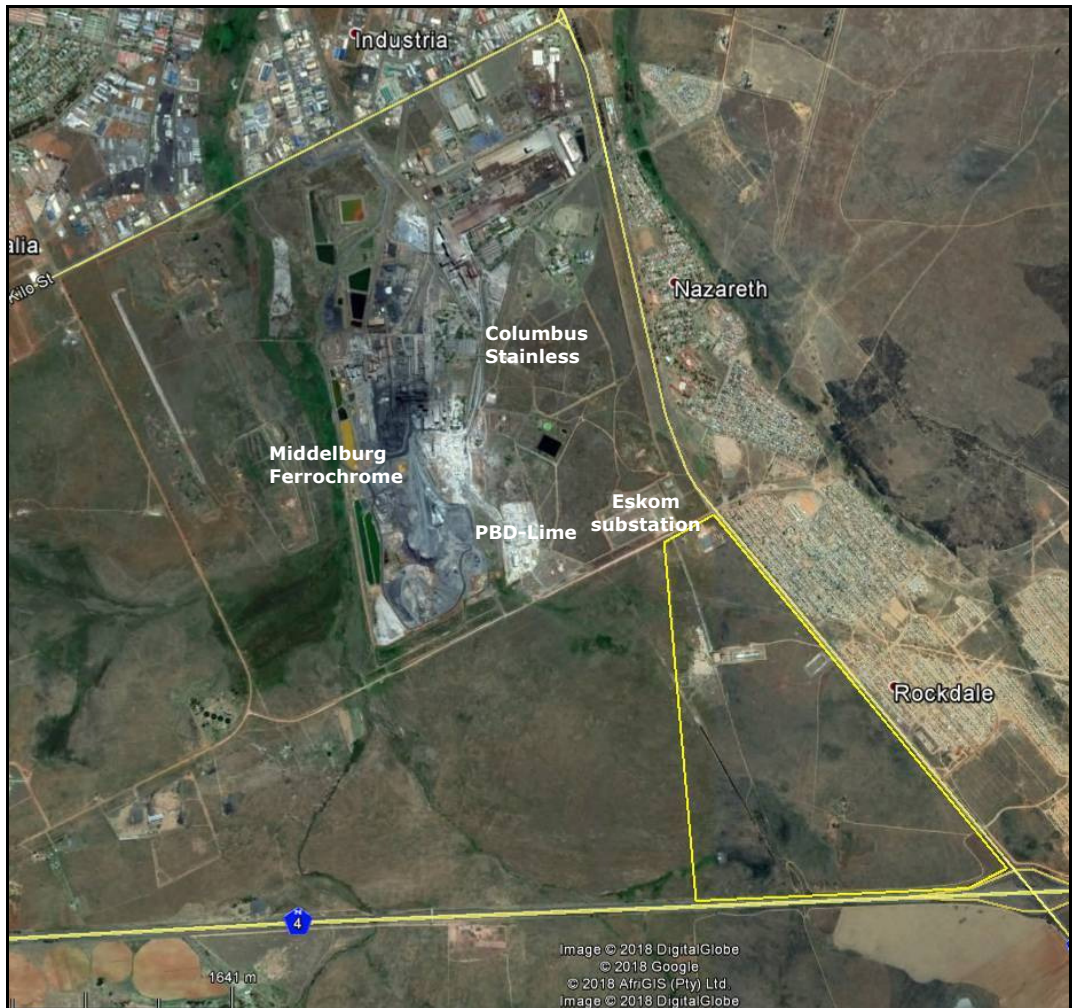
Figure 5.3a: An aerial view of Columbus Stainless and Middelburg Ferrochrome in relation to the said site.
