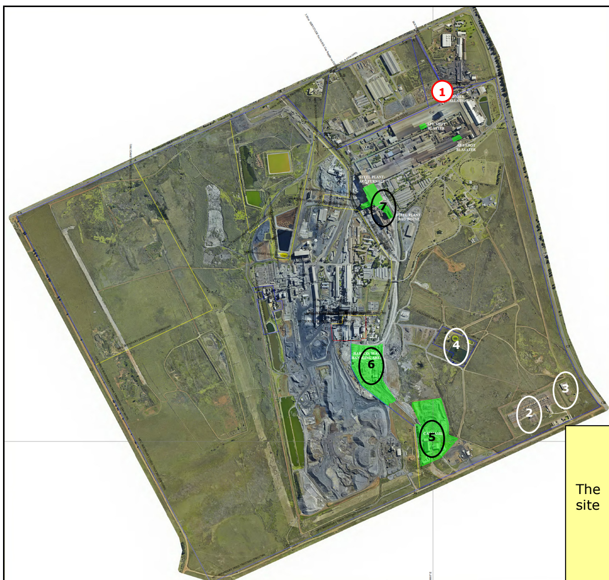
Figure 5.3b: An aerial view of the Columbus Stainless and Middelburg Ferrochrome facilities.
