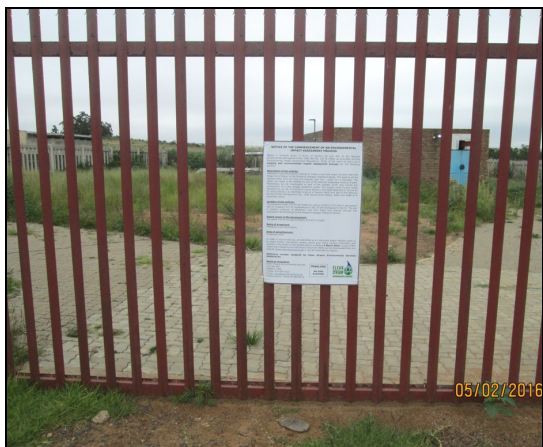
Photo 4.1: On-site notice at the Pine Ridge Pump Station (Point A)
