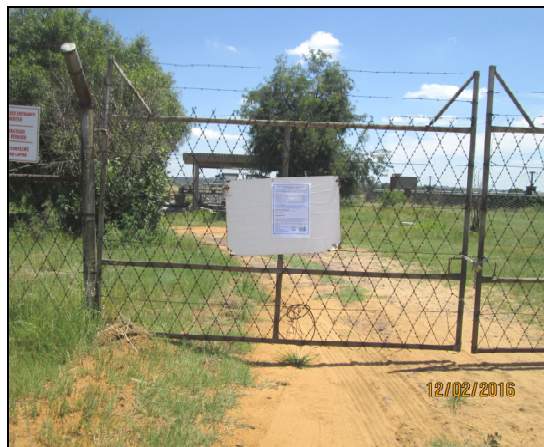
Photo 4.2: On-site notice at the Klipspruit Sewage Treatment Works (Point G)
