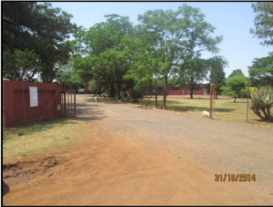
Photo 1: Main entrance and access road to site.
