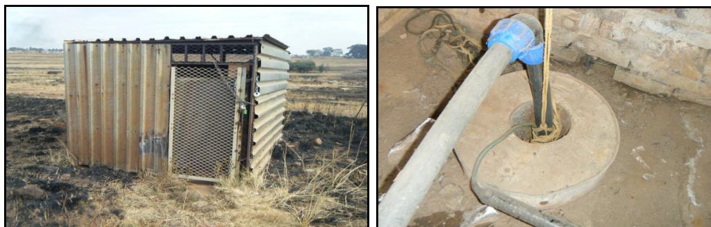
Figure 5.18: View of Borehole RDBM1 (taken from Gouws, 2014)
