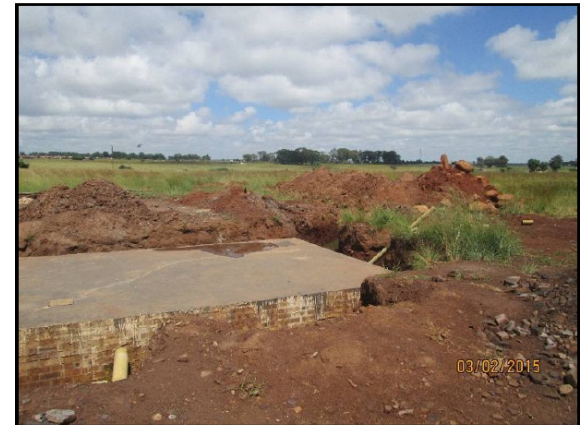
Photo 15: One of the new septic tanks on site.
