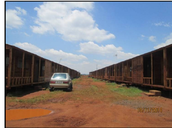
Photo 6: The new wooden structures
