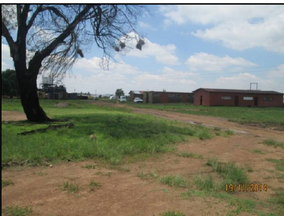
Photo 7: Another view of the new structures
