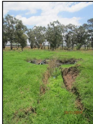
Photo 14: View of one of the old septic tanks on site.
