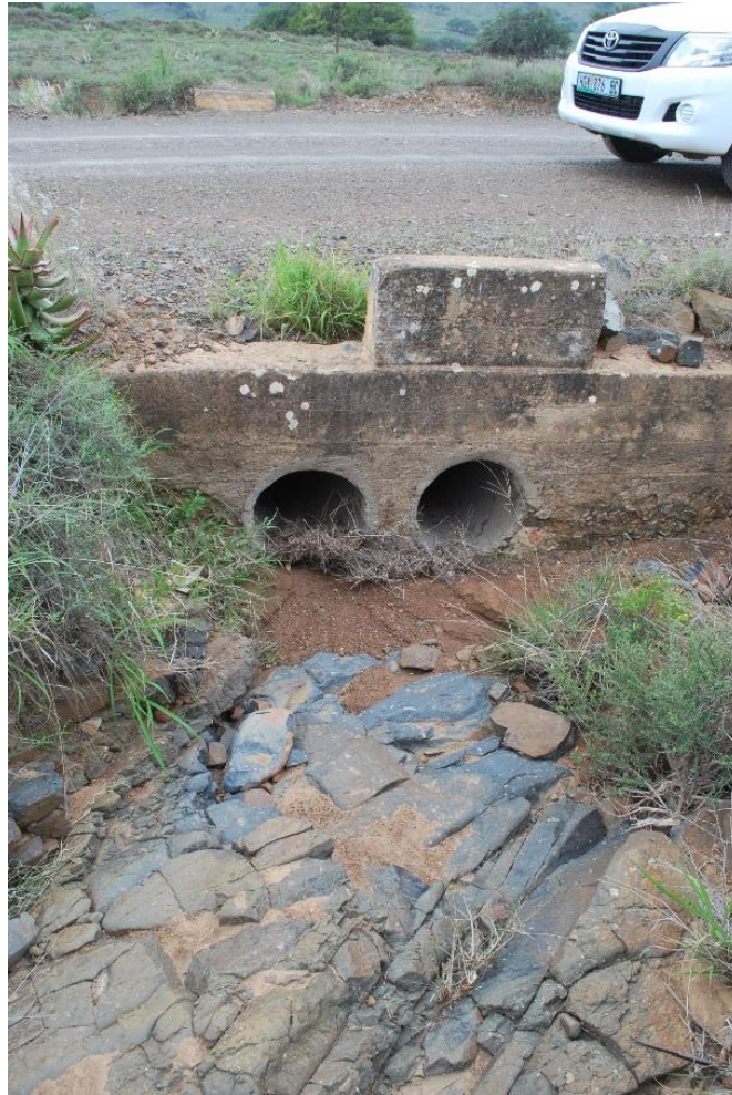
Plate 4: One of the main access roads with two small pipe culverts
