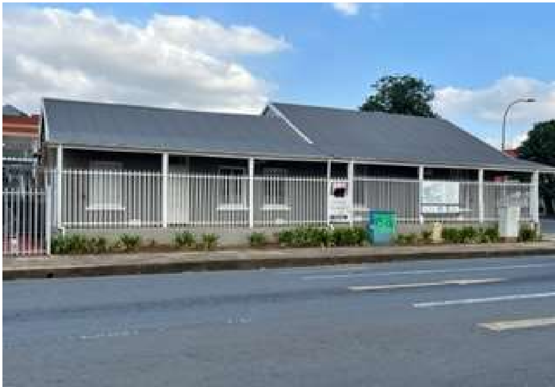
PHOTOGRAPH OF THE NORTH EAST ELEVATION OF THE BUILDING
