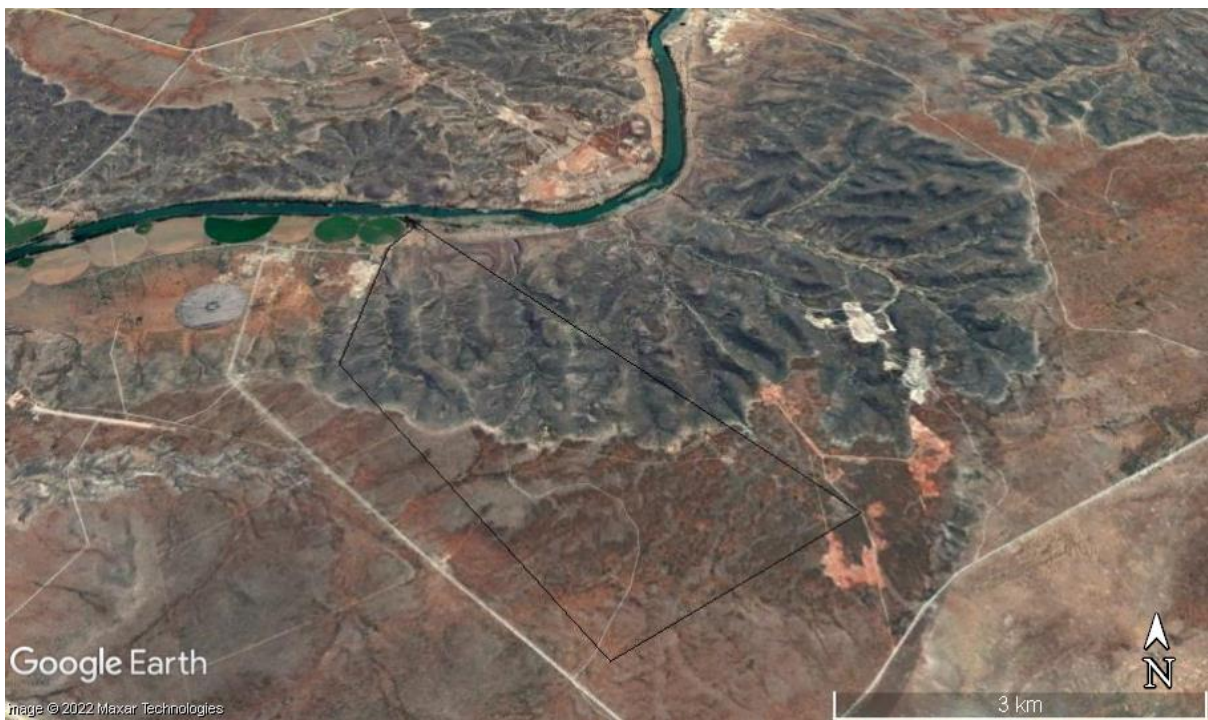
Figure 2: Google Earth Map of the proposed MRA on Portion 1 of Farm Saxondrift 20 with the section shown by the black outline.
