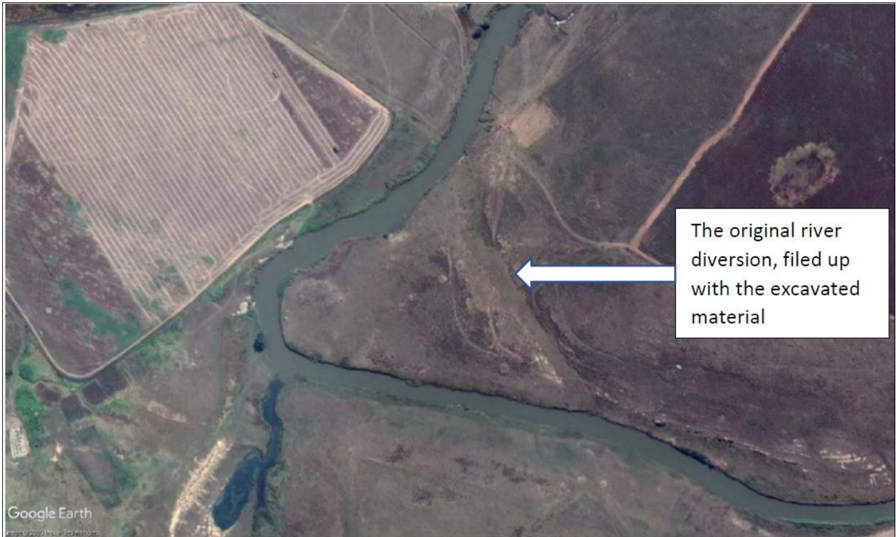
Figure 9:Original dug river diversion site
