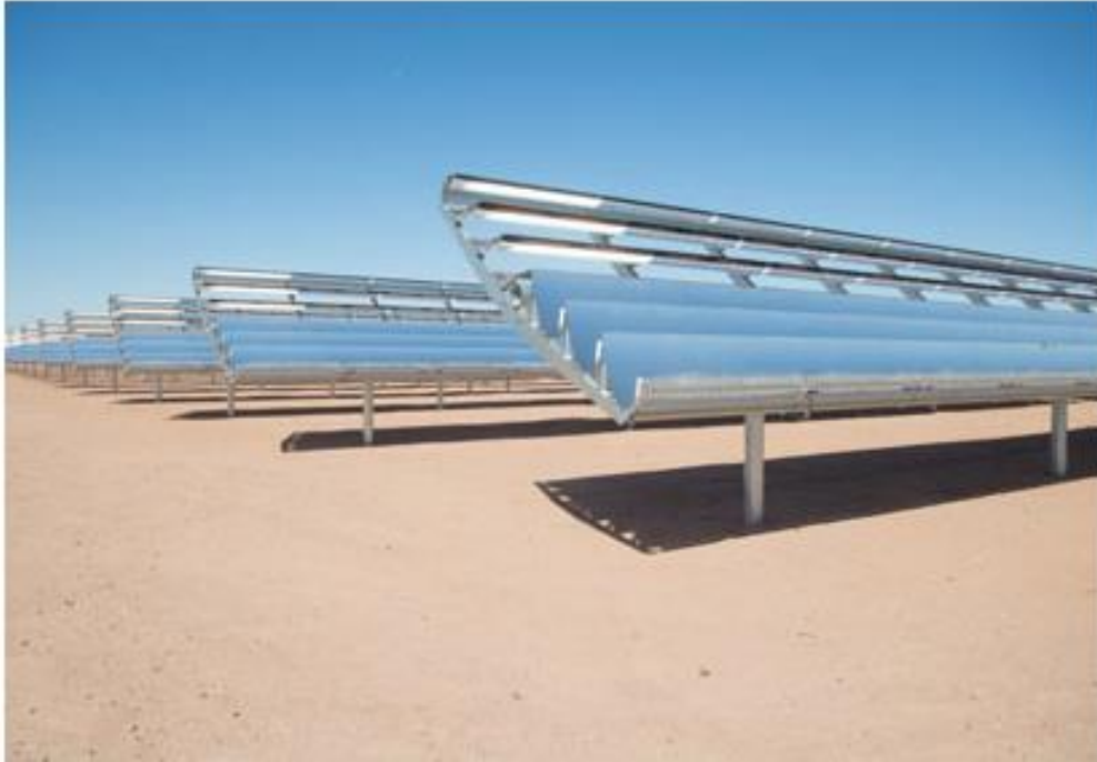
Figure 11 | CPV panel using optics to concentrate the sunlight (image courtesy of Mulilo)
