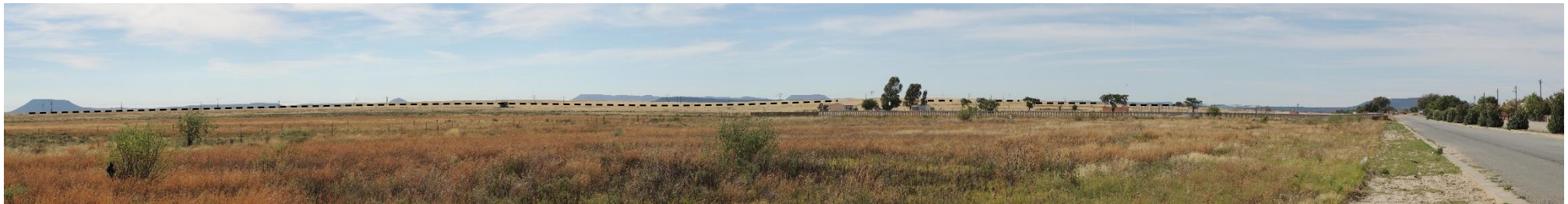
View east from Happy Valley towards proposed site with the approximate extent of the proposed project indicated in black
