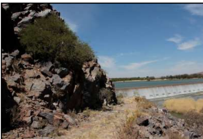
Figure 18. The Boegoeberg weir with DWA access track and koppie on the east side. The small green tree amongst the rocks is Boscia albitrunca .
