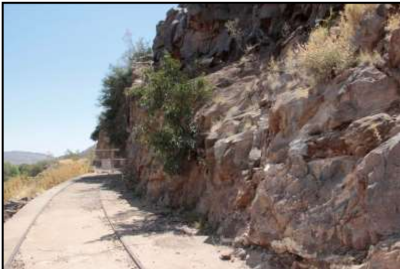
Figure 17. The DWA access road alongside the koppie at the Boegoeberg weir. Note the small Ficus cordata (Namaqua Rock Fig) on the rock face in the mid-ground.
