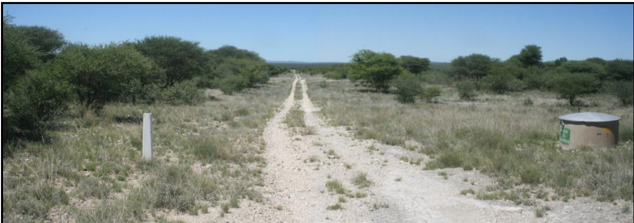
Figure 3: An access road already exist along the entire pipeline route. The structure on the right is an airvalve on the existing pipeline.
