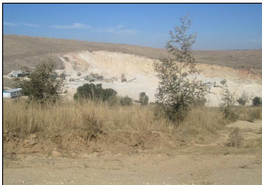
Photo 2.1: View of the quarry
