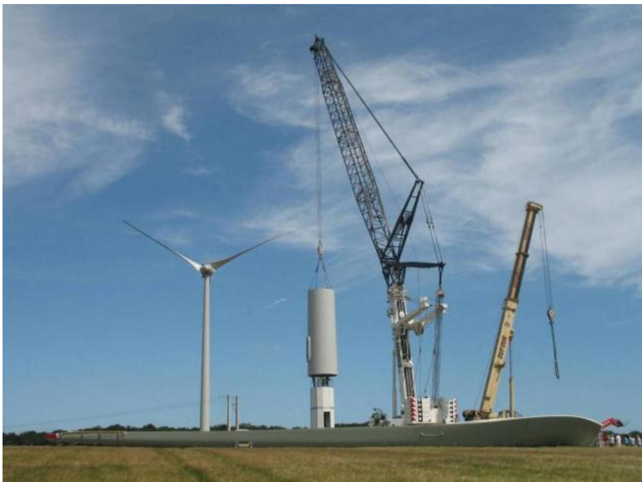
Figure 2-8: Assembly and erection of the tower sections using cranes.
