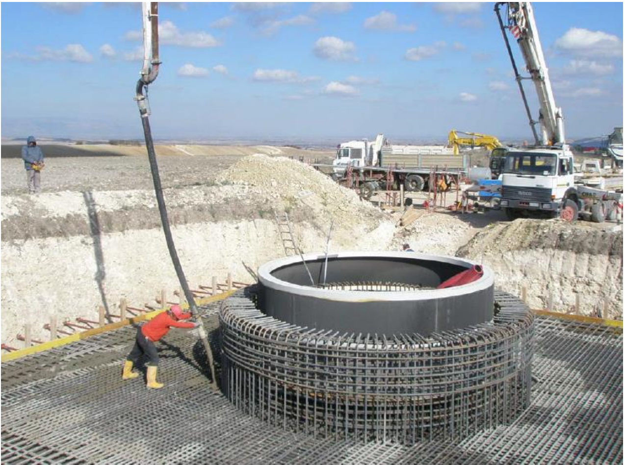
Figure 2-6: Concrete pouring of a turbine foundation – note the tower base collar in the foreground.
