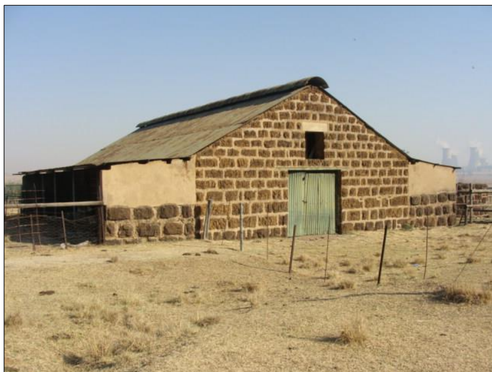
Figure 5.93: Outbuilding (wagon house) named site no. 16
