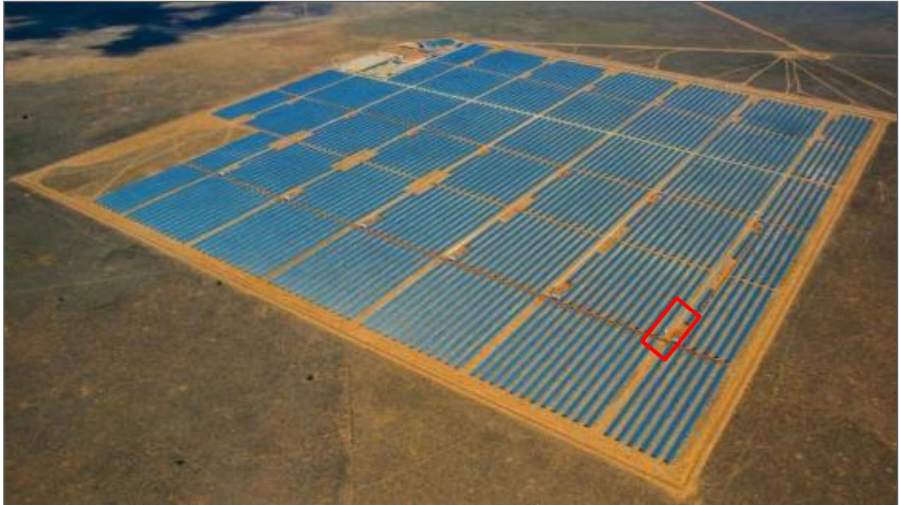
Figure 5-4: Inverter positioning on a PV panel array. The red block illustrates the location of an inverter within a PV panel array.
