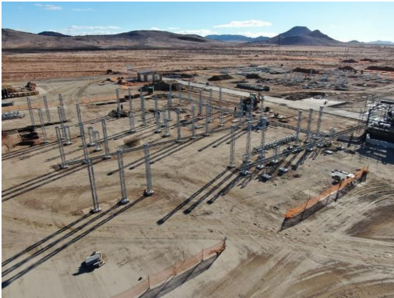
Figure 5-5: An IPP Substation under construction 23
