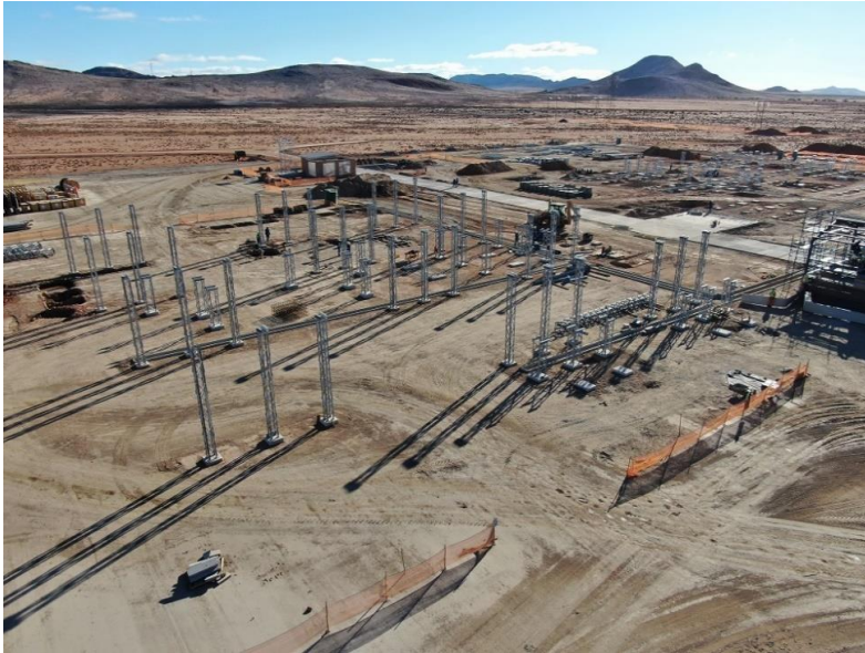
Figure 5-5: An IPP Substation under construction 23
