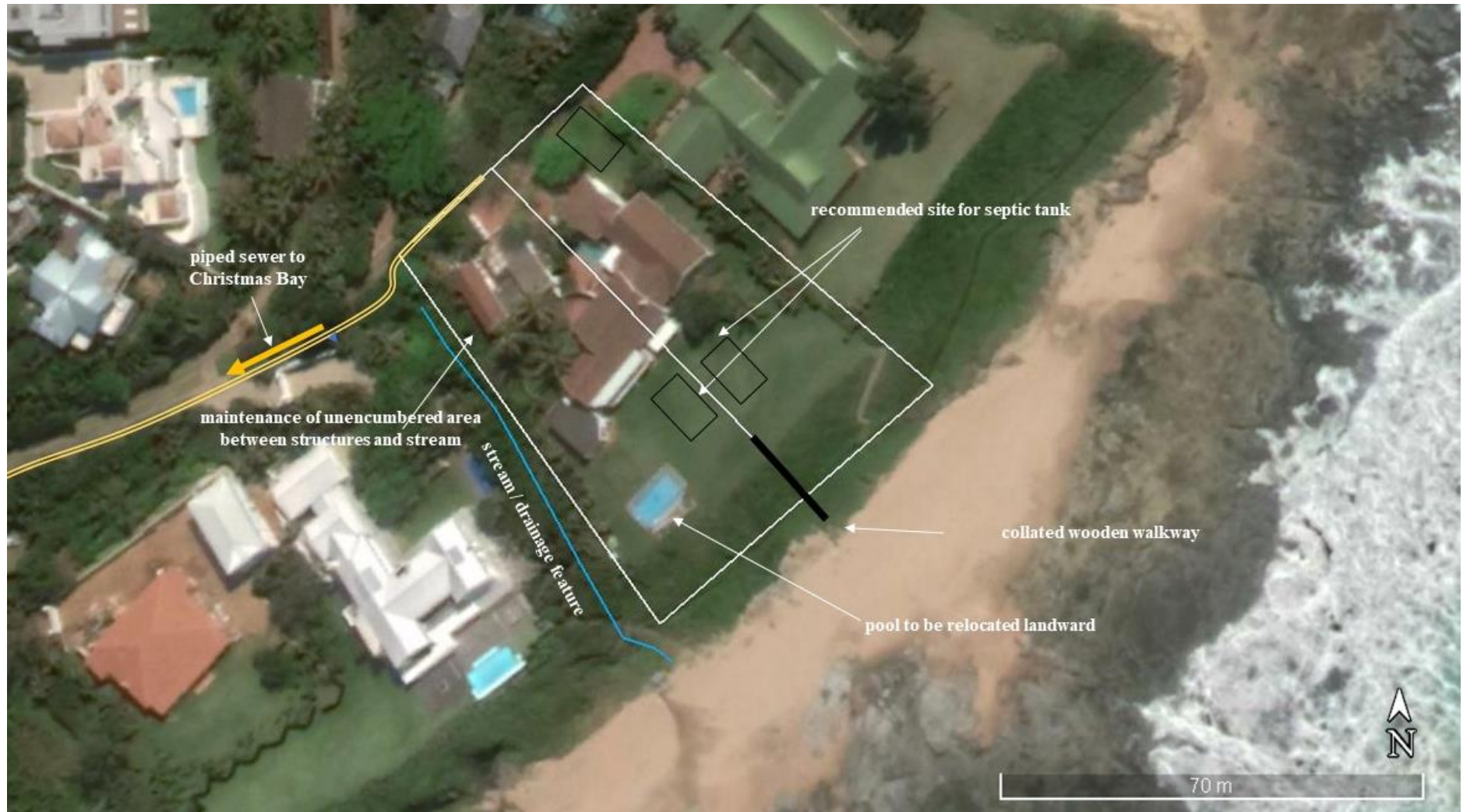
Figure 19. Aerial image indicating specific measures to be employed in respect of the proposed construction of homes at 99 Colwyn Drive. Note recommended evapo transpiration areas and alternative measures for disposal of sewerage to Christmas Bay.
