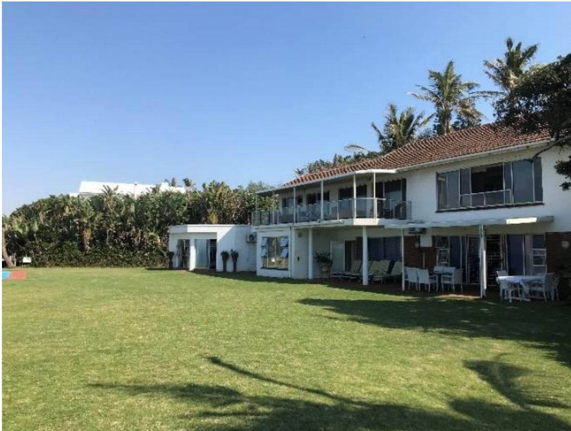
Figure 18. Image across subject site, showing structure to be demolished and lawn where septic tanks are to be situated.
