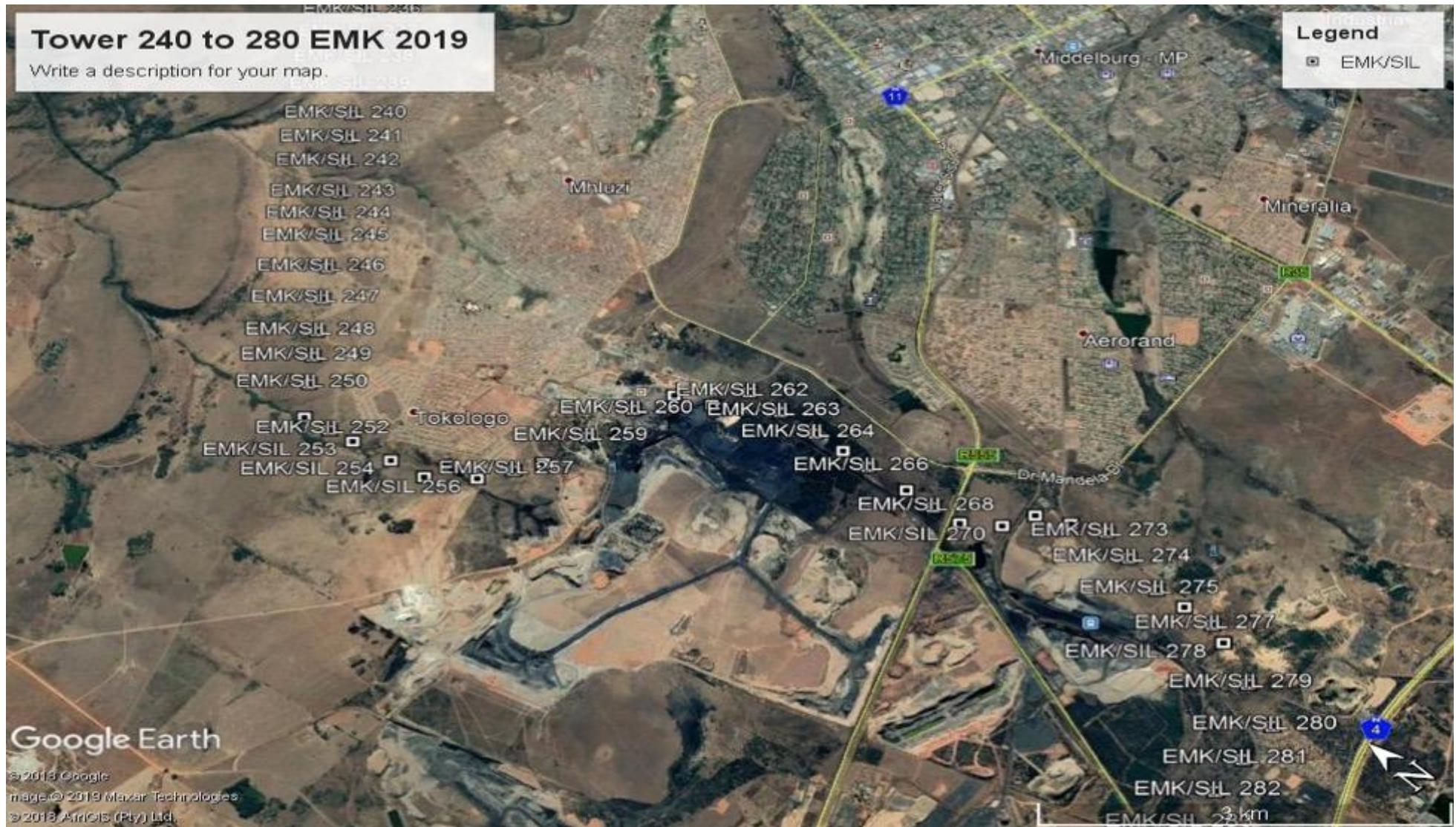
Figure 28: Powerline cuts through disturbed and built up area, all cutting through main roads R575 and R555
