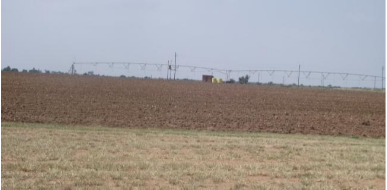
Figure 14: Pylon Structures 1 to 22 are located in predominantly commercial agriculture area characterised by commercial farming infrastructure
