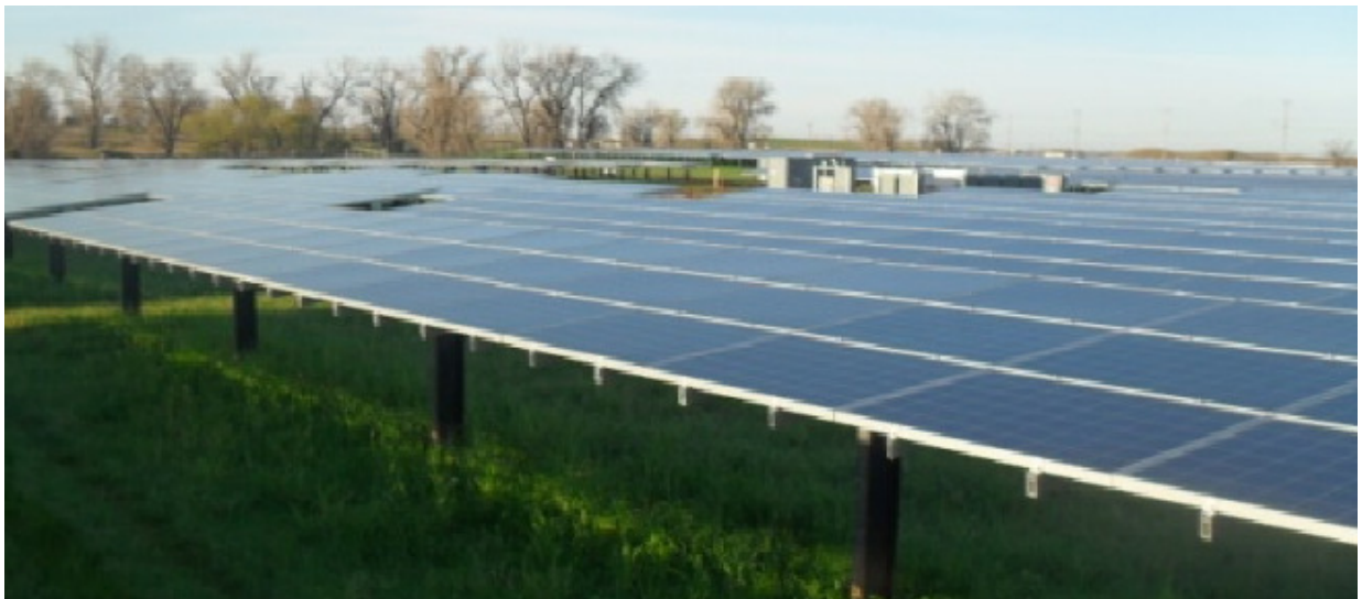
Figure 2 Frontal views of the PV arrays mounted on horizontal 1-axis tracker
