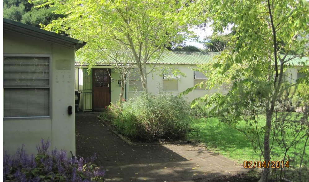
Prefabricated structures to be demolished.
