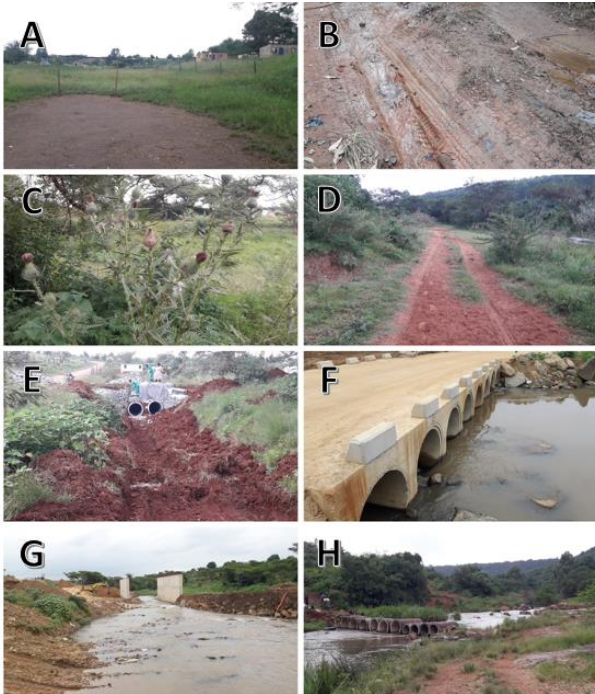
Figure 7-13 Impacts affecting the wetland health ratings. A) Compacted soccer field in drainage line. B) Preferential flow path over road causing erosion. C) Alien vegetation. D) Sediment sources. E) Excavation in drainage lines. F & H) Crossing structures. G) Diversion for construction on new bridge.
