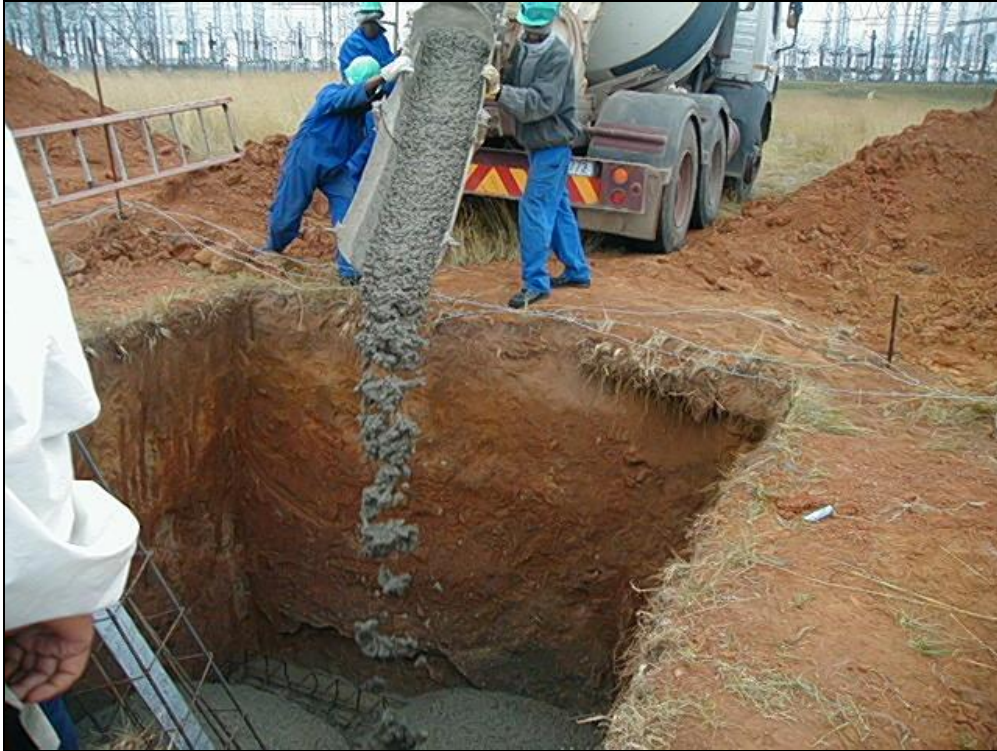
Plate 6: Construction of foundations for towers
