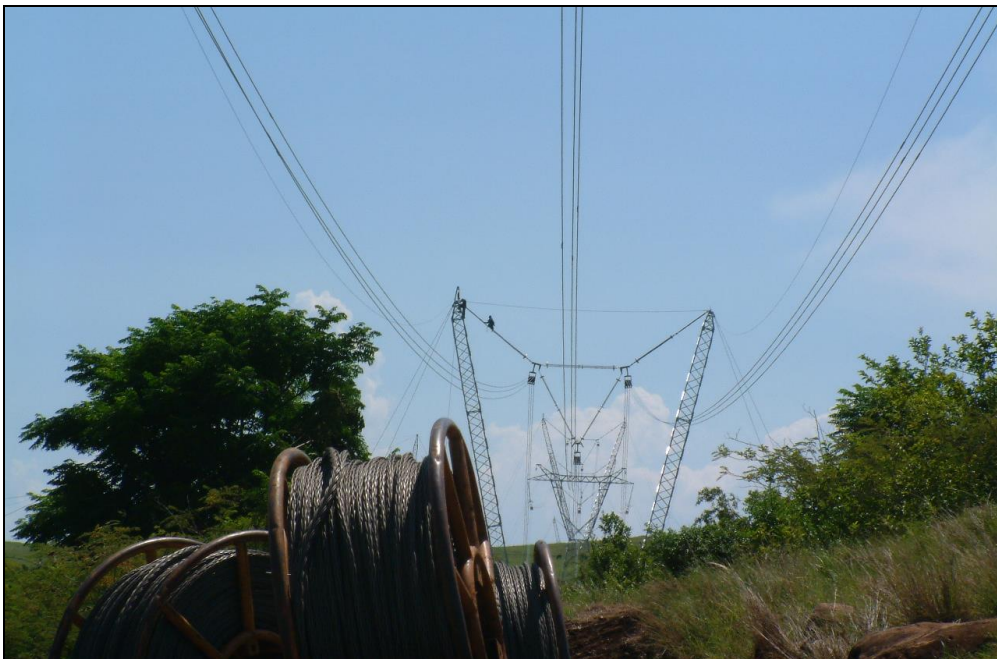
Plate 7: Guide wire being passed through towers
