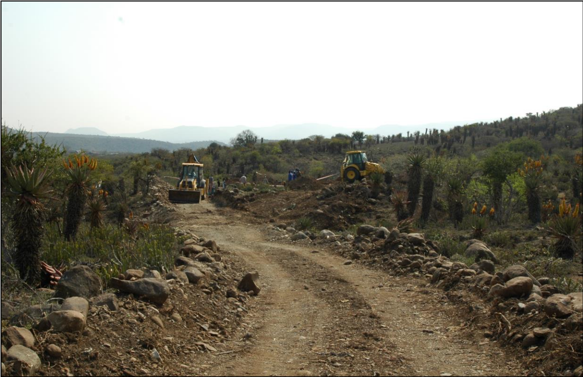
Plate 5: Construction/ upgrading access road
