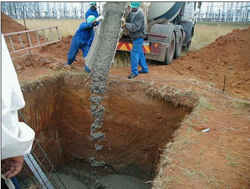
Plate 6: Construction of foundations for towers
