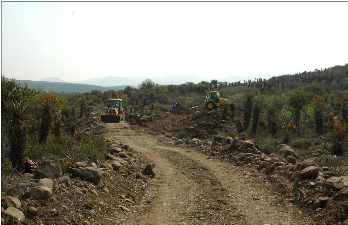
Plate 5: Construction/upgrading access road
