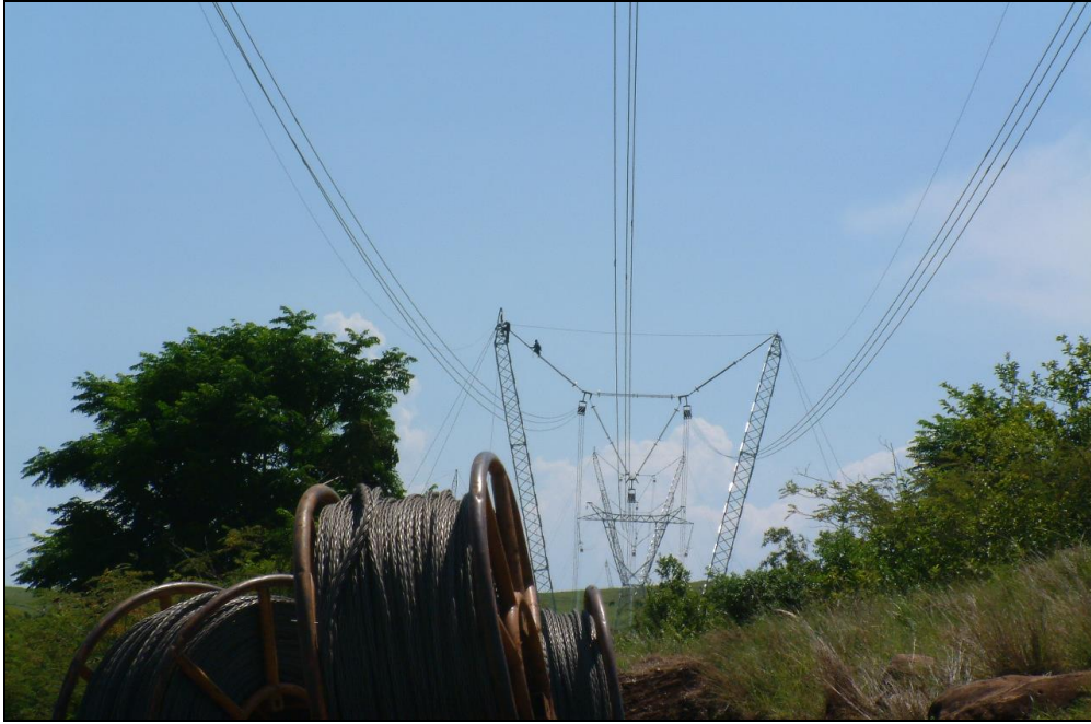
Plate 7: Guide wire being passed through towers
