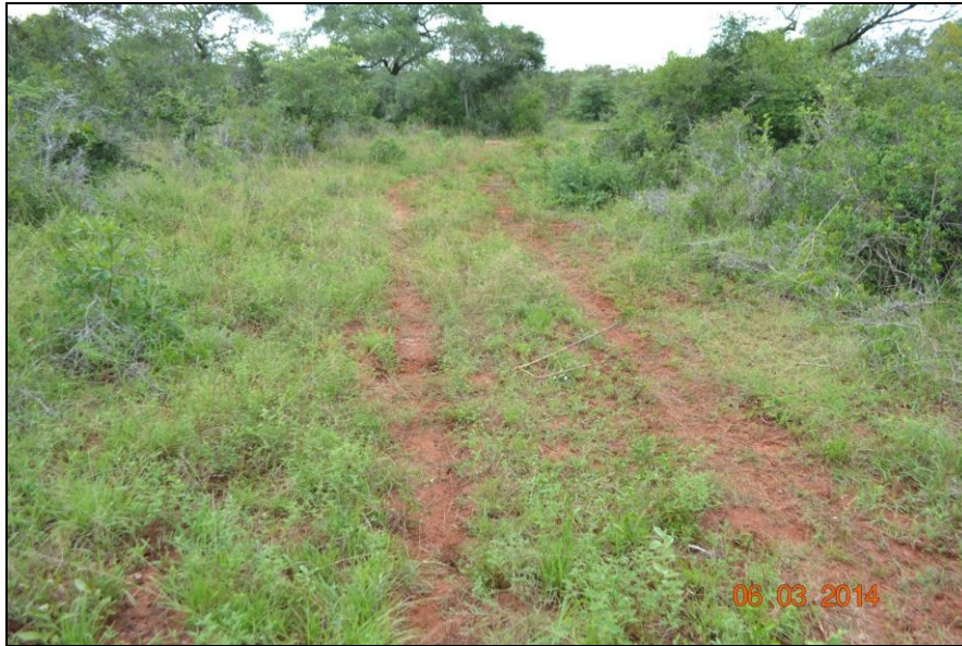
Plate 4: Bush cleared for vehicle access to tower sites
