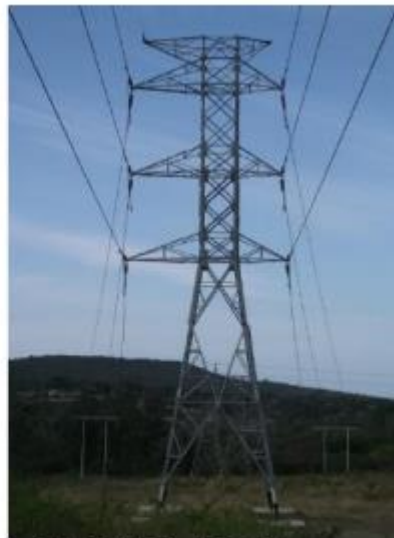
Plate 2: 245D Angle Strain Tower
