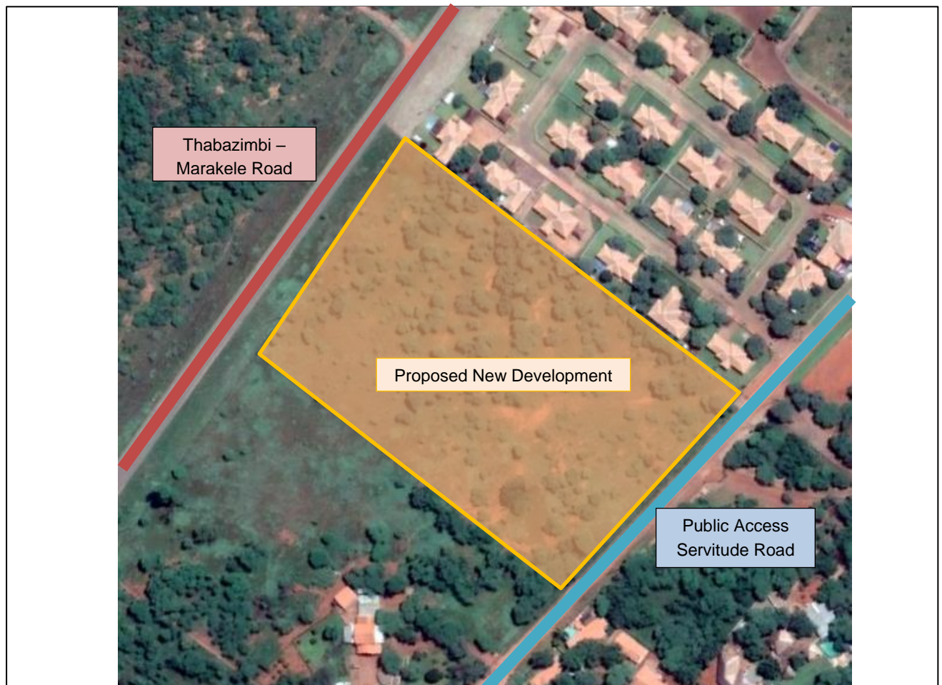
FIGURE 4-1: EXISTING ACCESS ROAD
