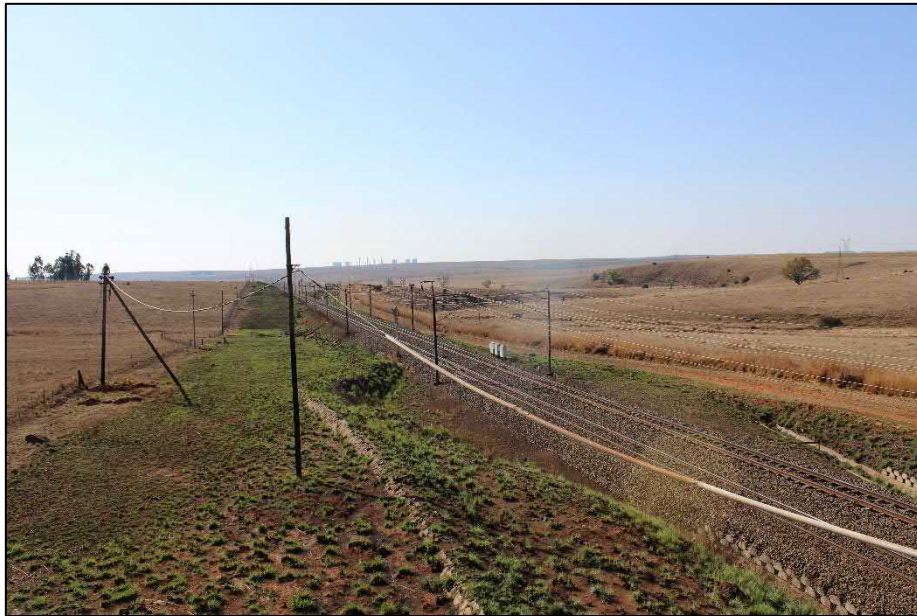
Figure 23: Rail infrastructure and power lines to the south-east of the Camden 1 SEF project area.
