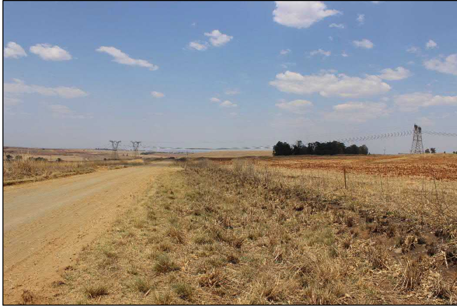
Figure 22: High voltage power lines feeding into Camden Power Station.
