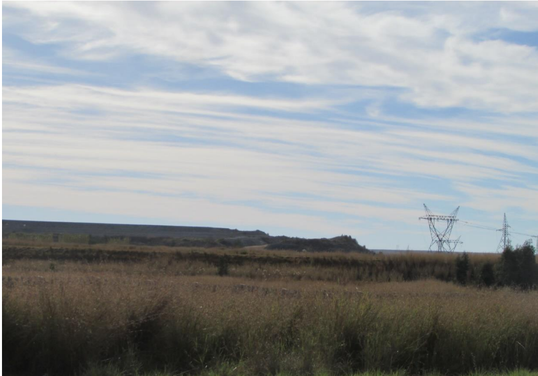
Figure 11: A view of the area with the Ash Discard Dump visible.
