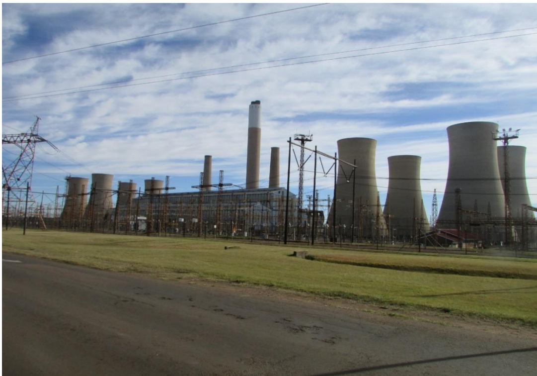
Figure 8: A view of the Komati Power Station.
