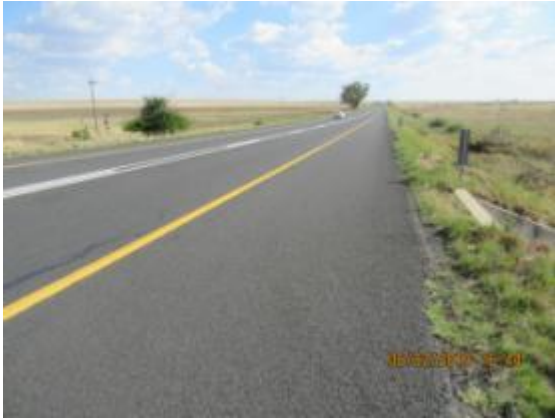
Figure 21 : View of the N1-16 road (South view)
