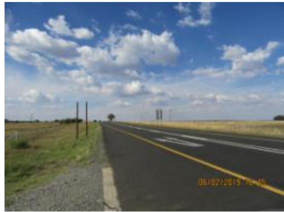
Figure 24: View of the N1-16 road (North view)
