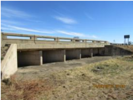
Figure 22: Bridge over Venterspruit
