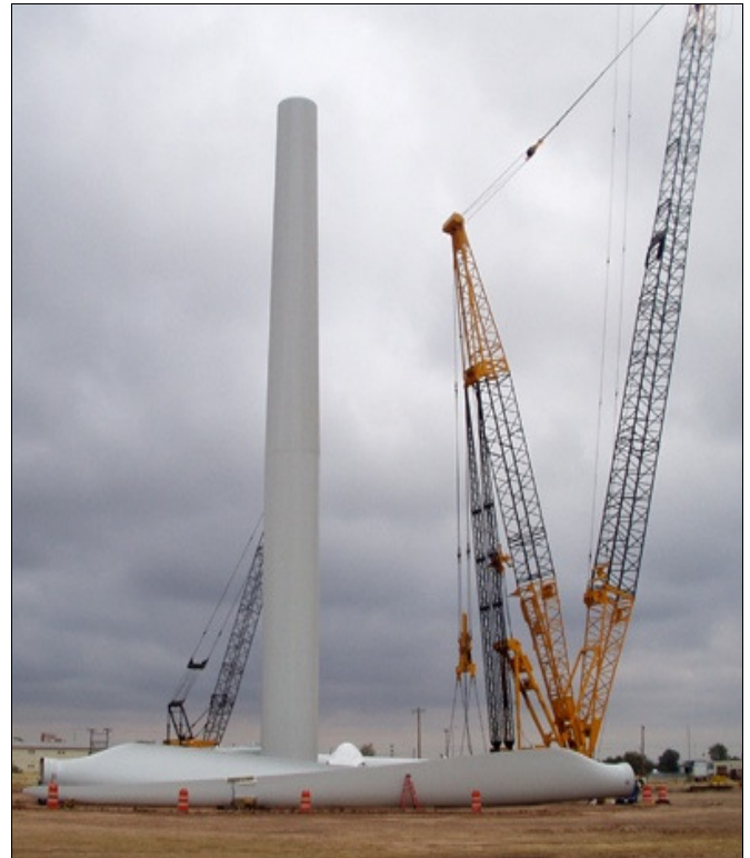
Figure 3. Wind Turbine Construction
