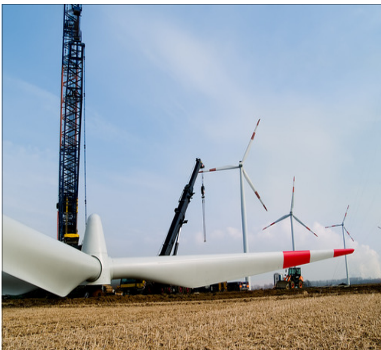
Figure 4. Wind Turbine Rotor and Blades during Assembly
