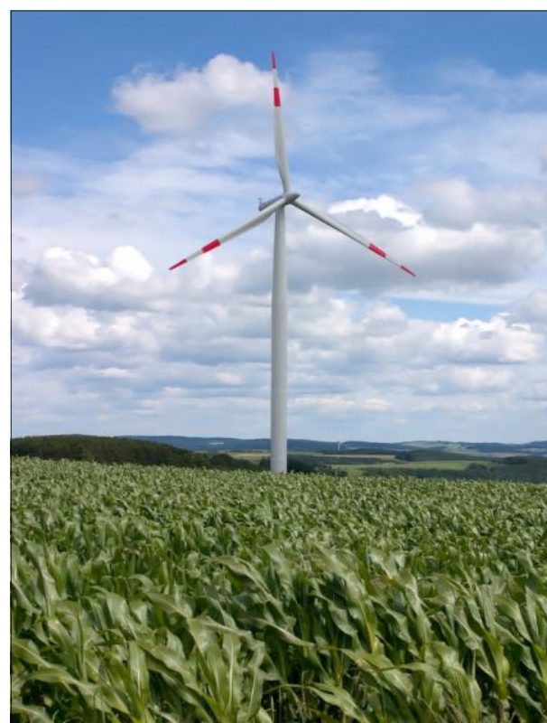
Figure 2. A Typical Wind Turbine
