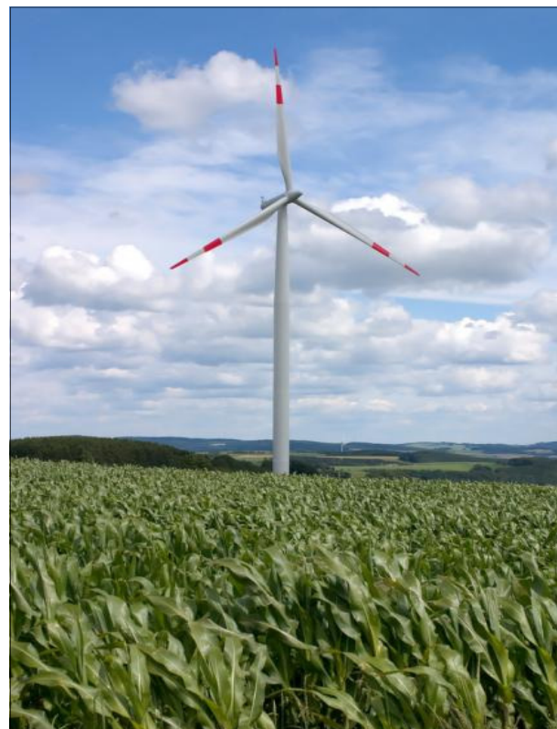
Figure 2. A Typical Wind Turbine
