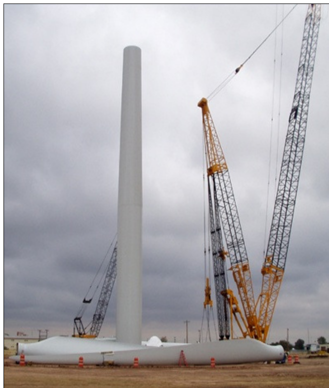
Figure 3. Wind Turbine Construction
