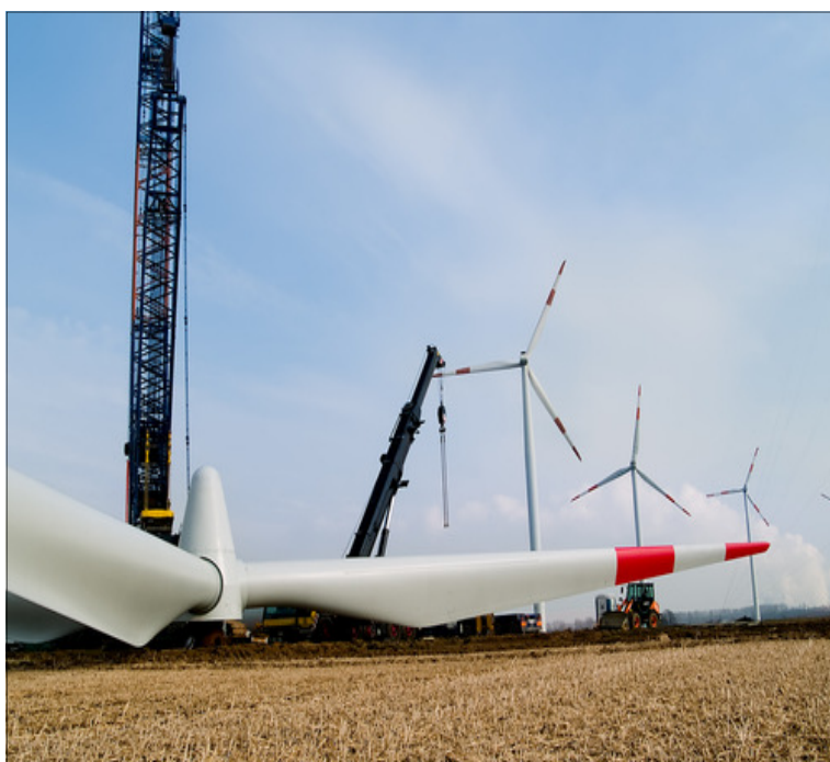
Figure 4. Wind Turbine Rotor and Blades during Assembly
