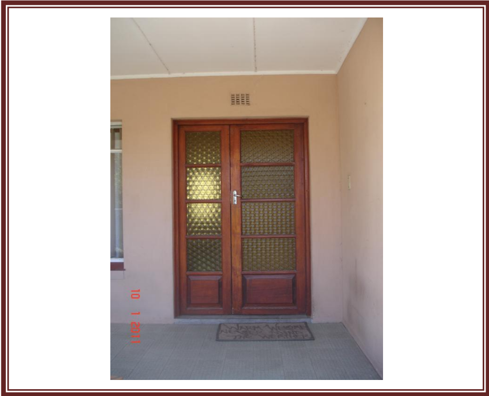
FRONT DOOR AND VERANDAH TILES
