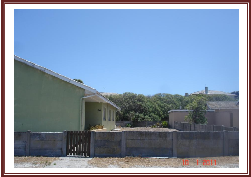
HOUSE 84 EAST FACE
