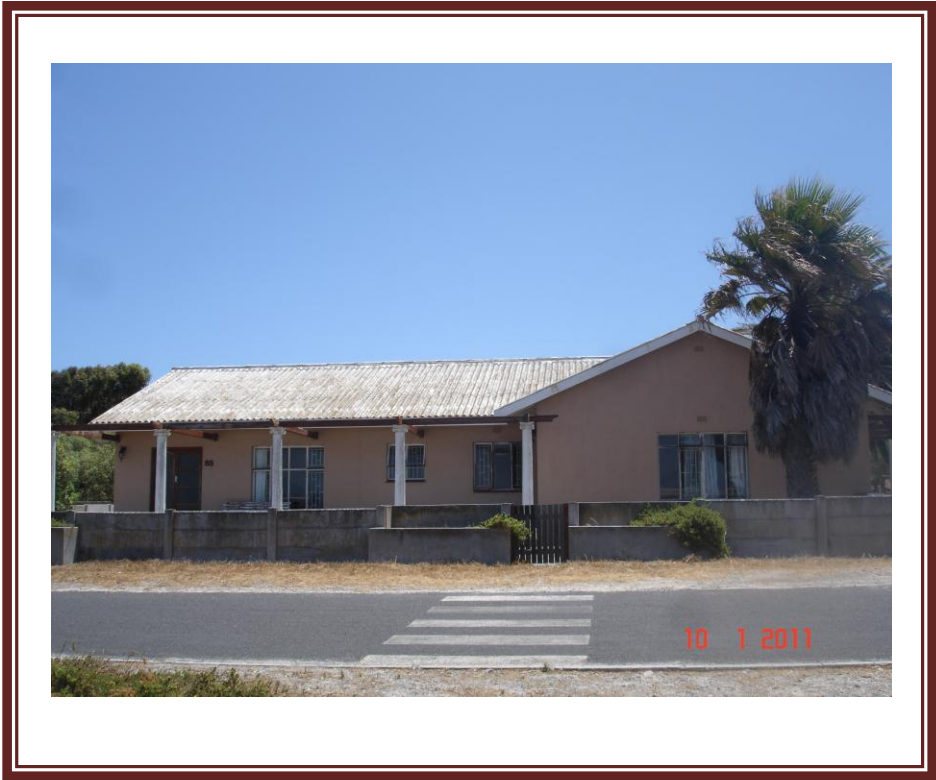
HOUSE 85 EAST FACE
