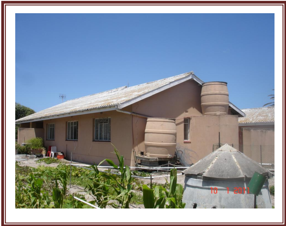
HOUSE 86 NW FACE
