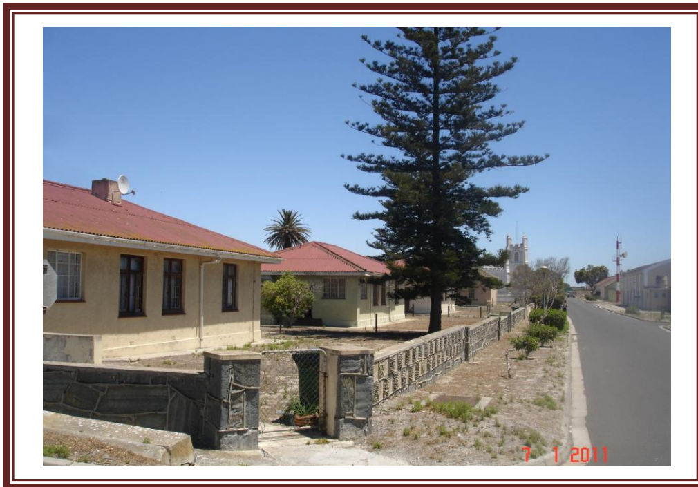
HOUSE 35 ENTRANCE AND STREETSCAPE WITH 36 AND 37 LOOKING NORTH
