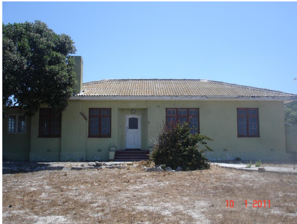
MAIN ENTRANCE FACING EAST
