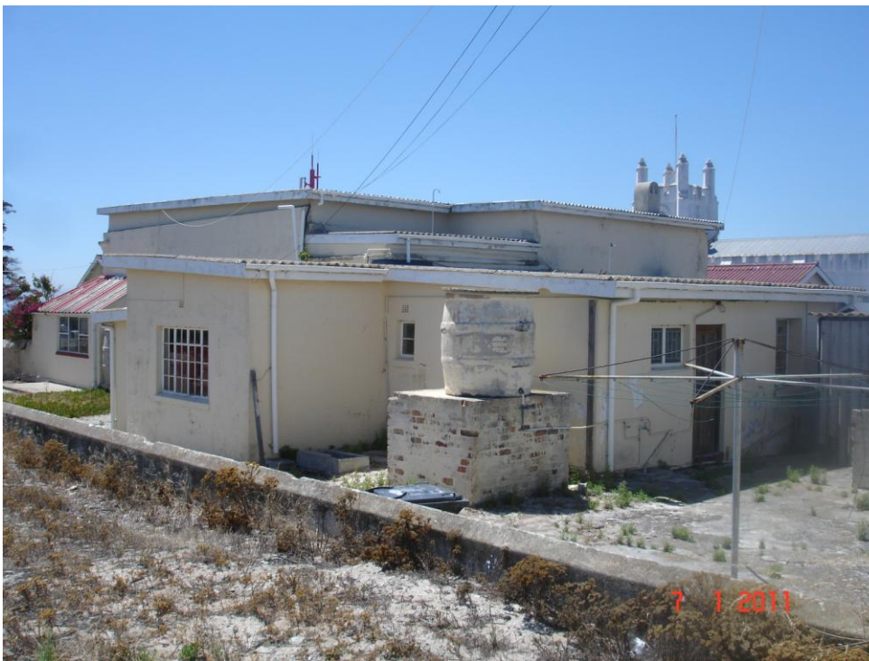
NW CORNER SHOWING ANNEXE
