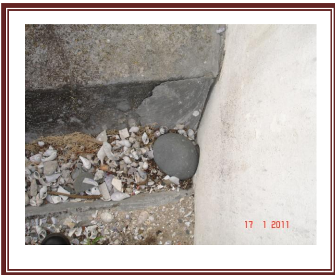
Fig.9.8. Large round stone blocking drainage SE corner
